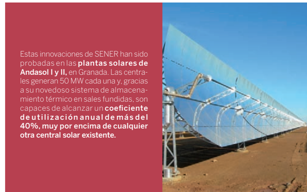
Colectores SENERtrough / SENERtrough collectors
